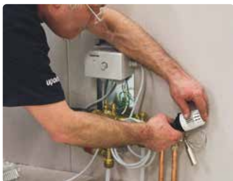
9. Montera termostatventilen.
